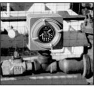
the Swichgage instrument monitors the entire lead line, sensing any blockage whether sludge build-up in the line or an accidental closed valve. The pressure trans- mitter threads into a 2 NPT tee on the lead line.
